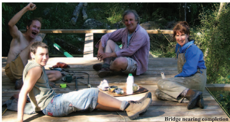
Bridge nearing completion
